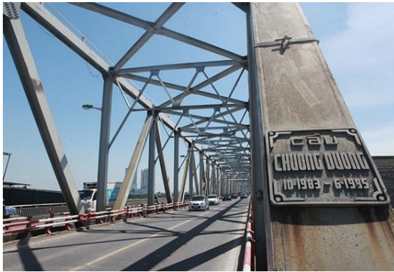
Fig.1 – Chuong Duong bridge (Vietnam)
