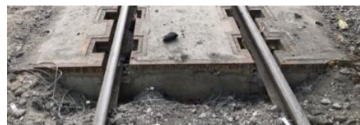
Fig. 4 - Set up for strain gauges on the slab at the site
