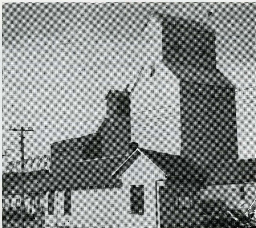
Newly Erected Grain Elevator
