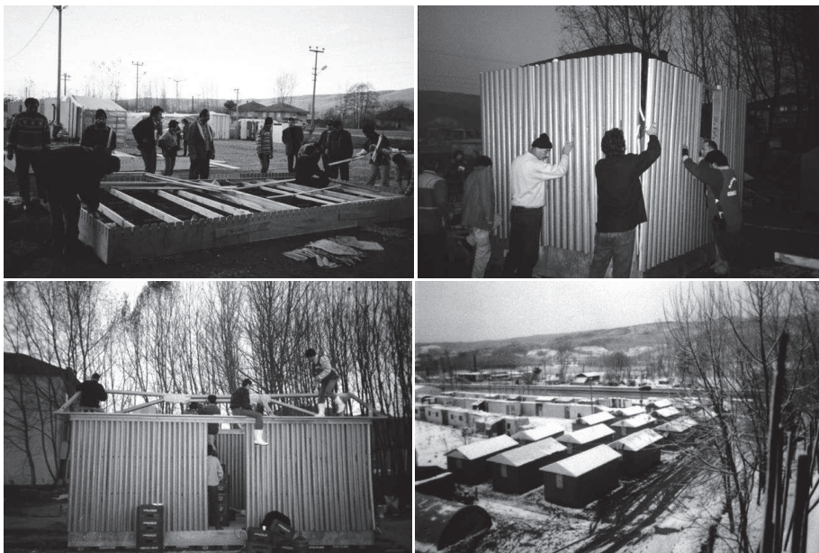
Figure 2 – Kit solutions: assembly process by local community and cluster of the Paper Log Houses designed by Shigeru Ban (source: https://archnet.org )
