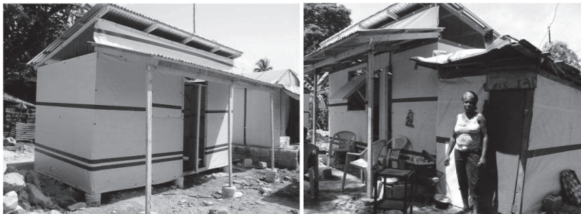
Figure 3 – Units modifications: temporary housing unit before being used and after the user modifies it (source: http://openarchitecturenetwork.org ).
