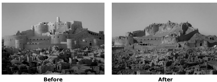
Figure 3 – Bam citadel before and after the 2003 earthquake.
