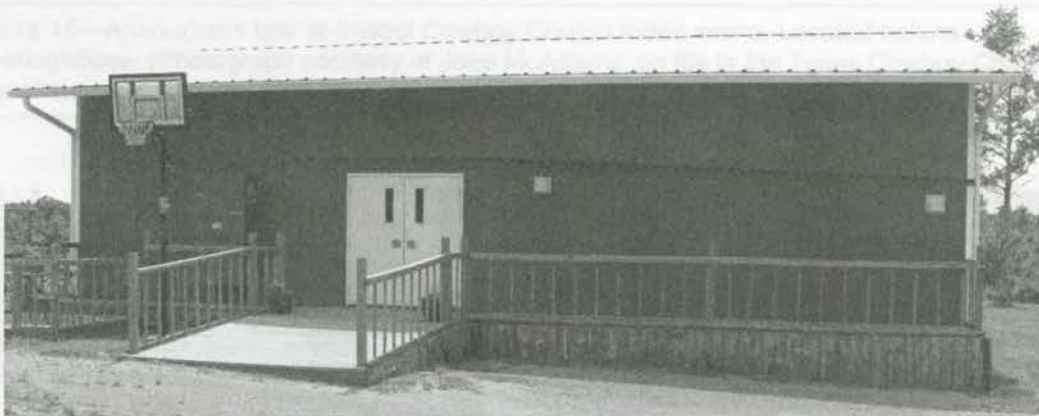
Figure 13—Impact Cowboy Church classroom building located behind meetinghouse. (Photograph courtesy of Jake McAdams; on file in the Texas Cowboy Church Oral Histories collection, ETRC.)
