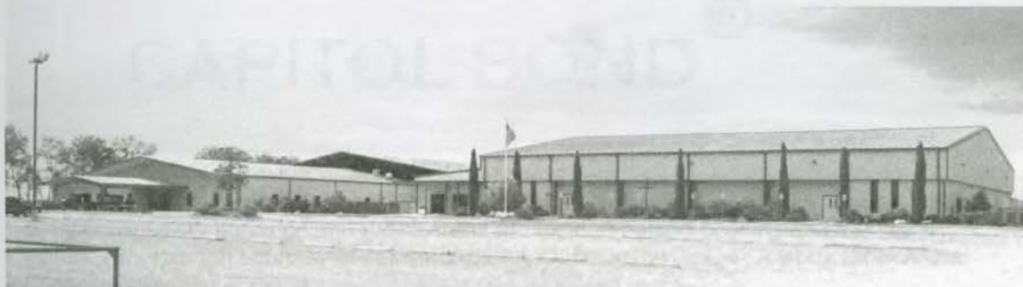
Figure 2—Front view of the The Cowboy Church of Ellis County campus at the junction of Interstate 35 E and Highway 287 in Waxahachie, Texas. The rodeo arena is located behind the left-hand building. (Photograph courtesy of Jake McAdams; on file in the Texas Cowboy Church Oral Histories collection, ETRC.)
