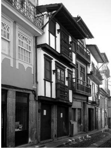
Figure 1 – Rua Nova's house, the former seat of Guimarães GTL.
