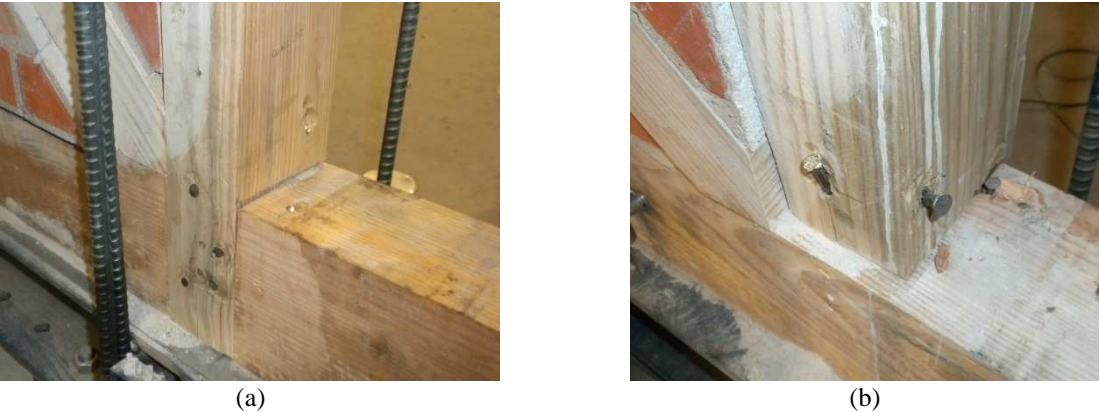
Figure 6. Additional nails inserted at bottom connections
