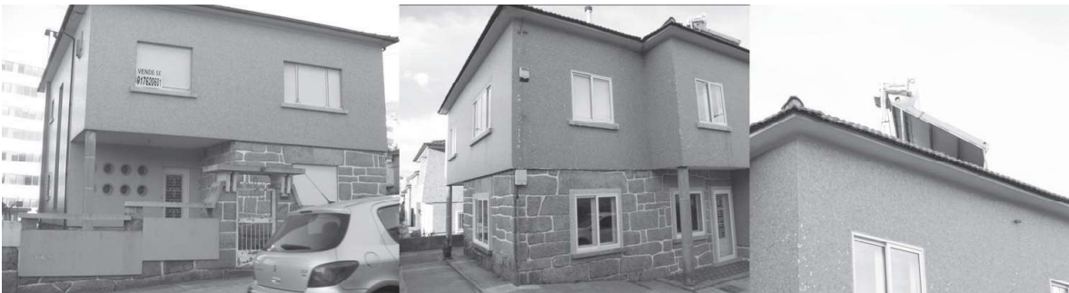
Figure 4: Images of the building after and before refurbishment
