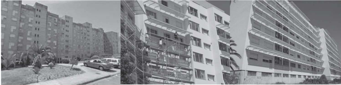
Figure 3. Images of the building after and before refurbishment.
