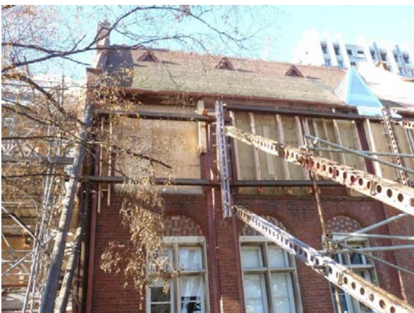
Figure 10: Shoring of the West wall
