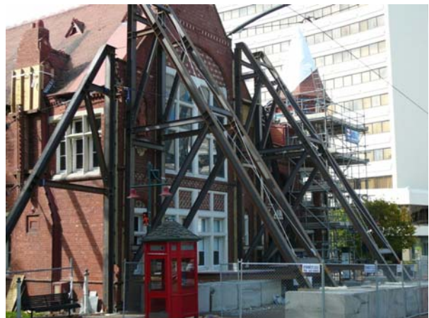
Figure 6: Shoring of the South wall
