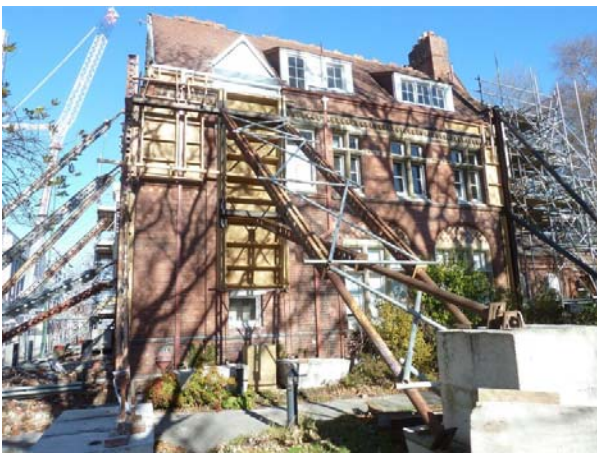
Figure 9: Shoring of the North wall
