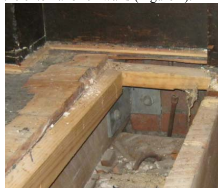
Figure 2: Typical floor ties to wall
