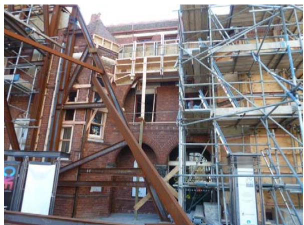
Figure 7: Shoring of the South wall in the entryway
