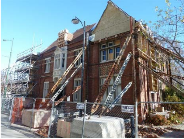
Figure 8: Shoring of the East wall
