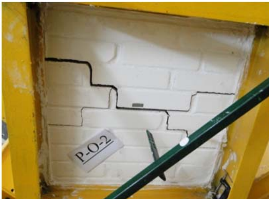
Fig. 4. Typical failure under two-way, out-of-plane bending of wall panels
