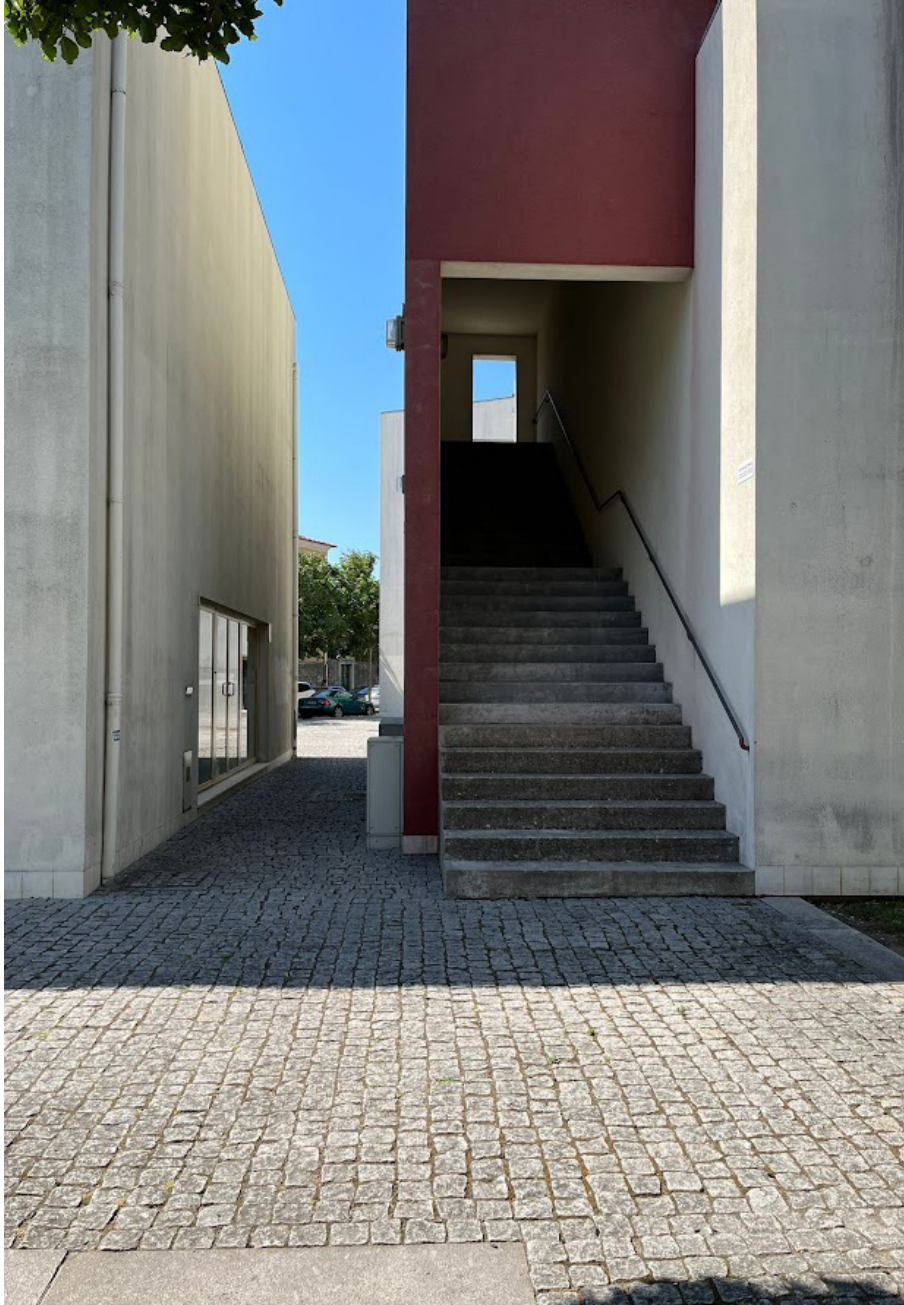
Figure 3.2.6. Photograph taken in Bouça neighbourhood. Focus in the exterior circulation stairs.
