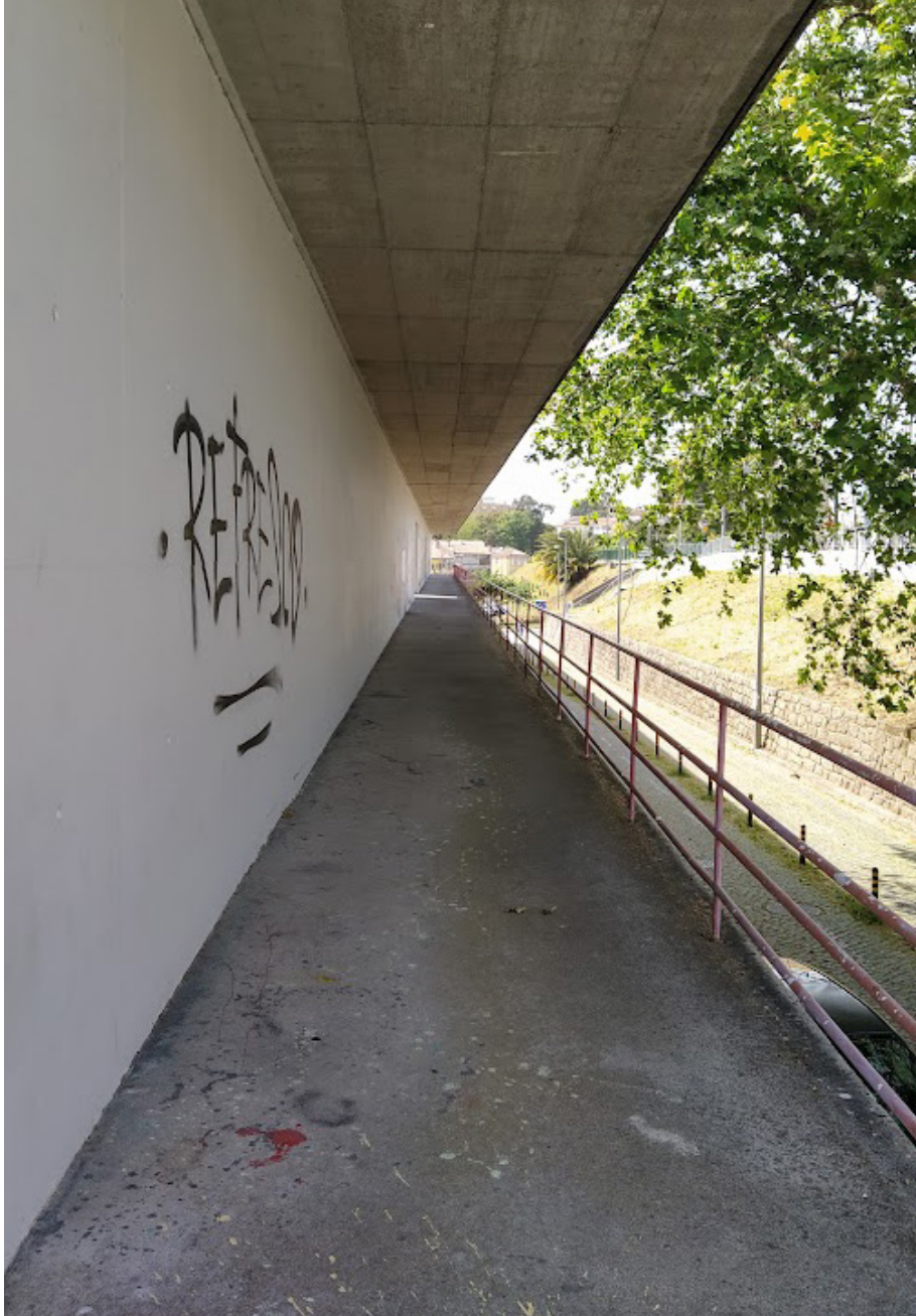
Figure 3.2.7. Photograph taken in Bouça neighbourhood. Circulation concrete wall.
