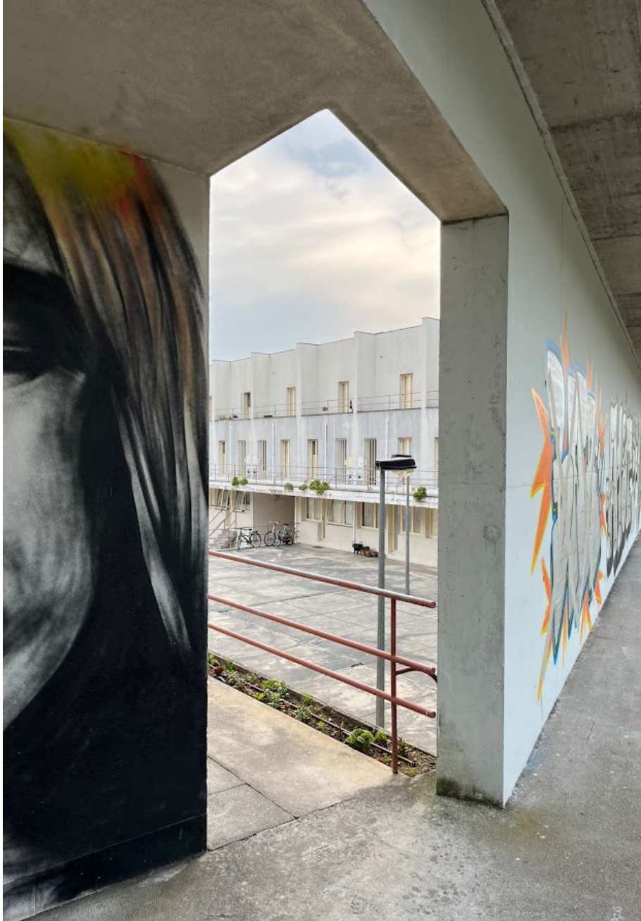
Figure 3.2.9. Photograph taken in Bouça neighbourhood. Passage through the concrete wall on the third floor.
