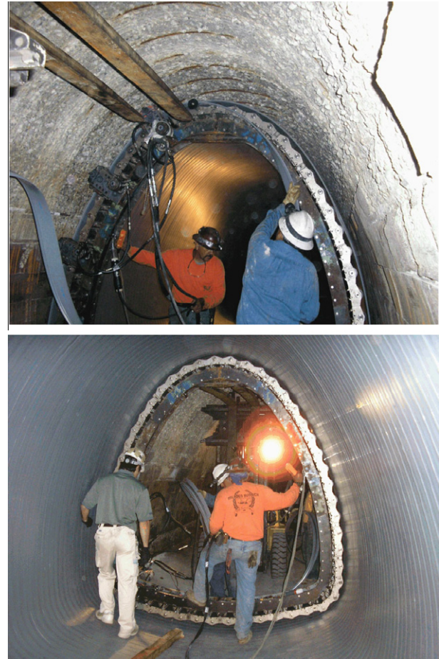
Fig. 7. Rehabilitation of a reinforced concrete pipeline sewer with a PVC liner.
