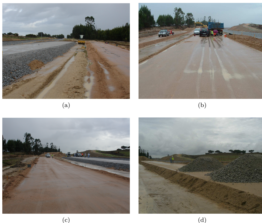
Figure 4.7: ETRE : (a) SC layer; (b) CA31.5 material over SC layer; (c) and (d) general overview of SC and CA31.5 trial layers
