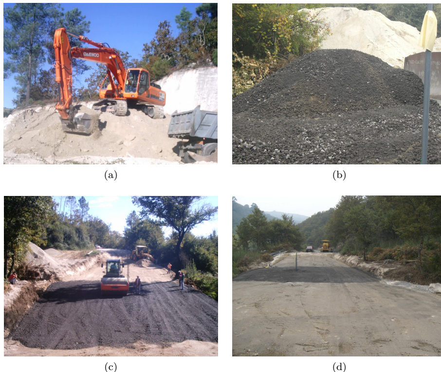
Figure 4.10: FTRE : (a) SP material; (b) ISAC material; (c) and (d) general overview of SC and ISAC trial layers
