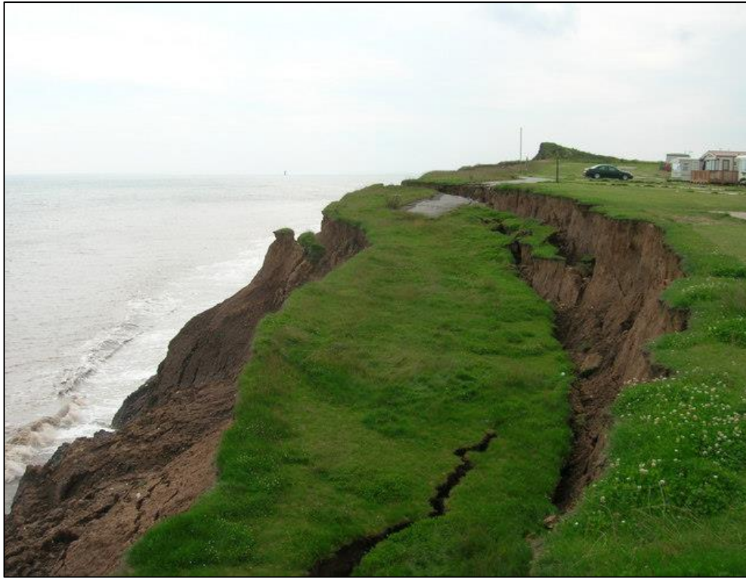
Figure 11: A photograph taken in 2009 of the coastal erosion at Aldbrough (JThomas, 2009).
