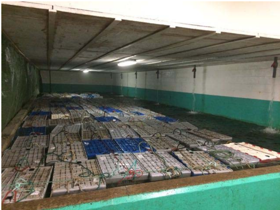
Figure 1.10 Typical shore-side reception reservoir system in the Homarus americanus fishery with a flow-through ambient seawater supply and supplemental aeration (Clearwater Seafoods LP photo).
