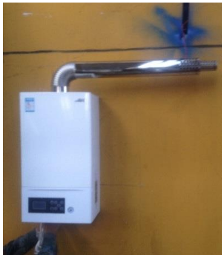
Fig. 5- 14: Image of the selected gas boiler
