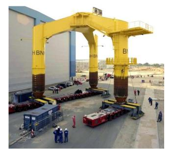
Figure 2-32 – Tri-pile Foundation (Brickwell, 2012)
