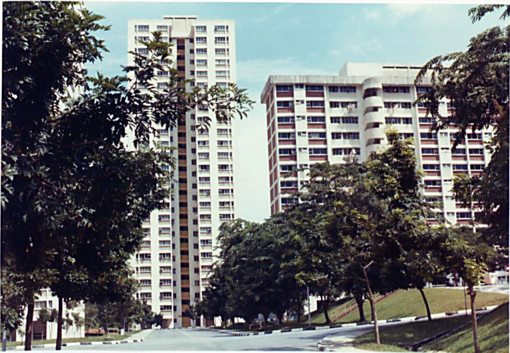
Photo 4: These blocks of middle-income flats at Farrer Court were built by the HUDC in the mid-1970s
