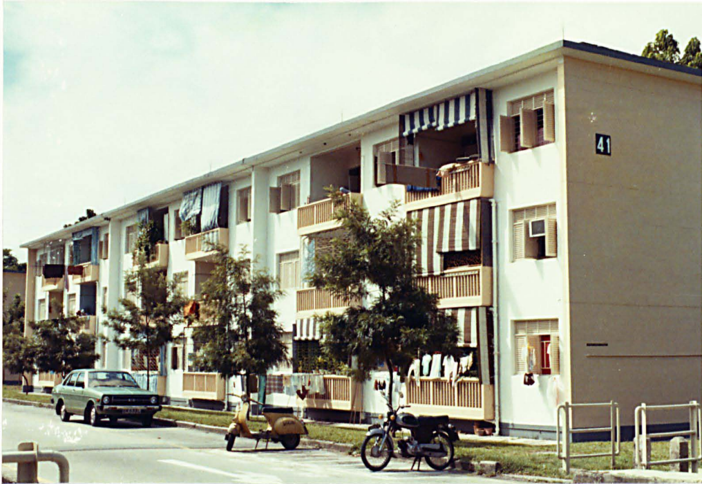
Photo 5: This block of low-rise flats at Prince Charles Crescent was constructed by the SIT in the early 1950s
