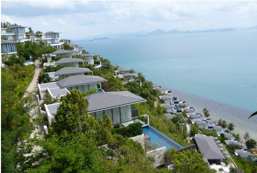
Figure 5.22: Encroachment on the mountain in sub district Taling Ngam
