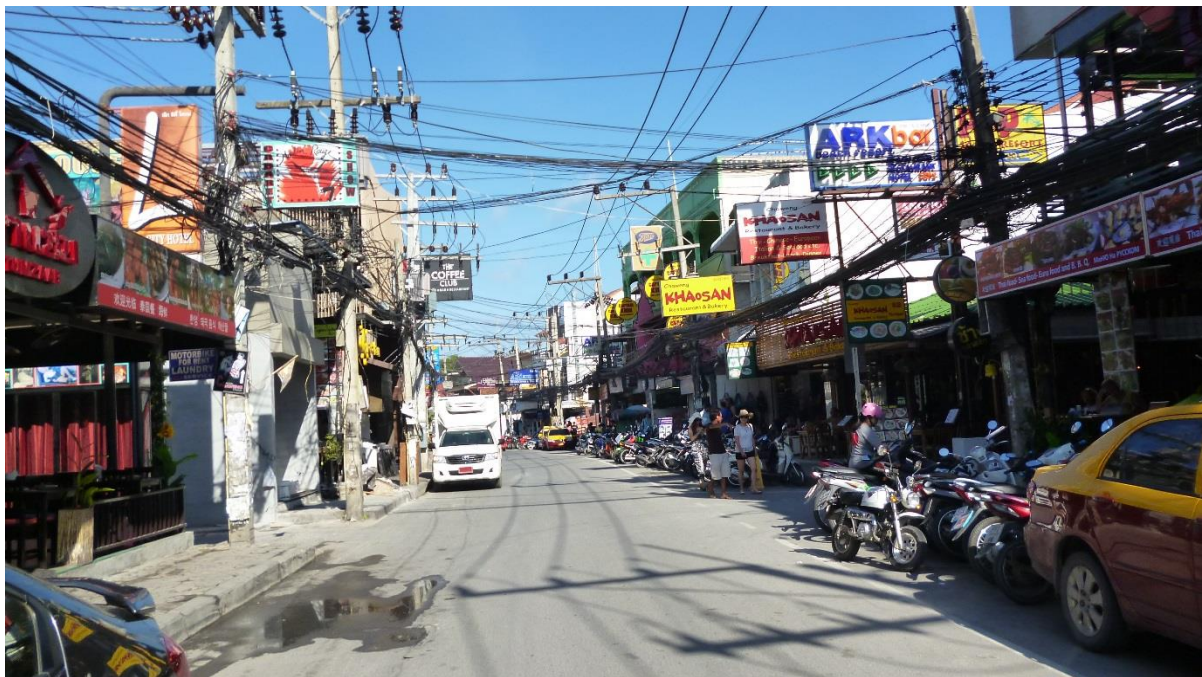
Figure 5.8: Unplanned Development in Chaweng beach, Bo Phud
