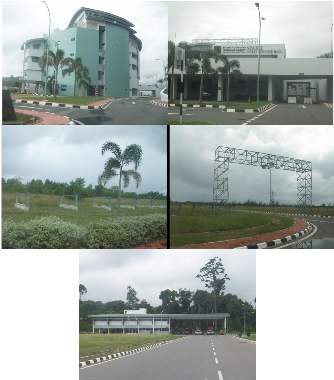
Figure 8 Facilities and infrastructures at SPARK [From top left to bottom: SPARK Centre; Multipurpose Hall, cable connectors (1); cable connectors (2); and SPARK Fire Department Source: Fieldwork, 2012
