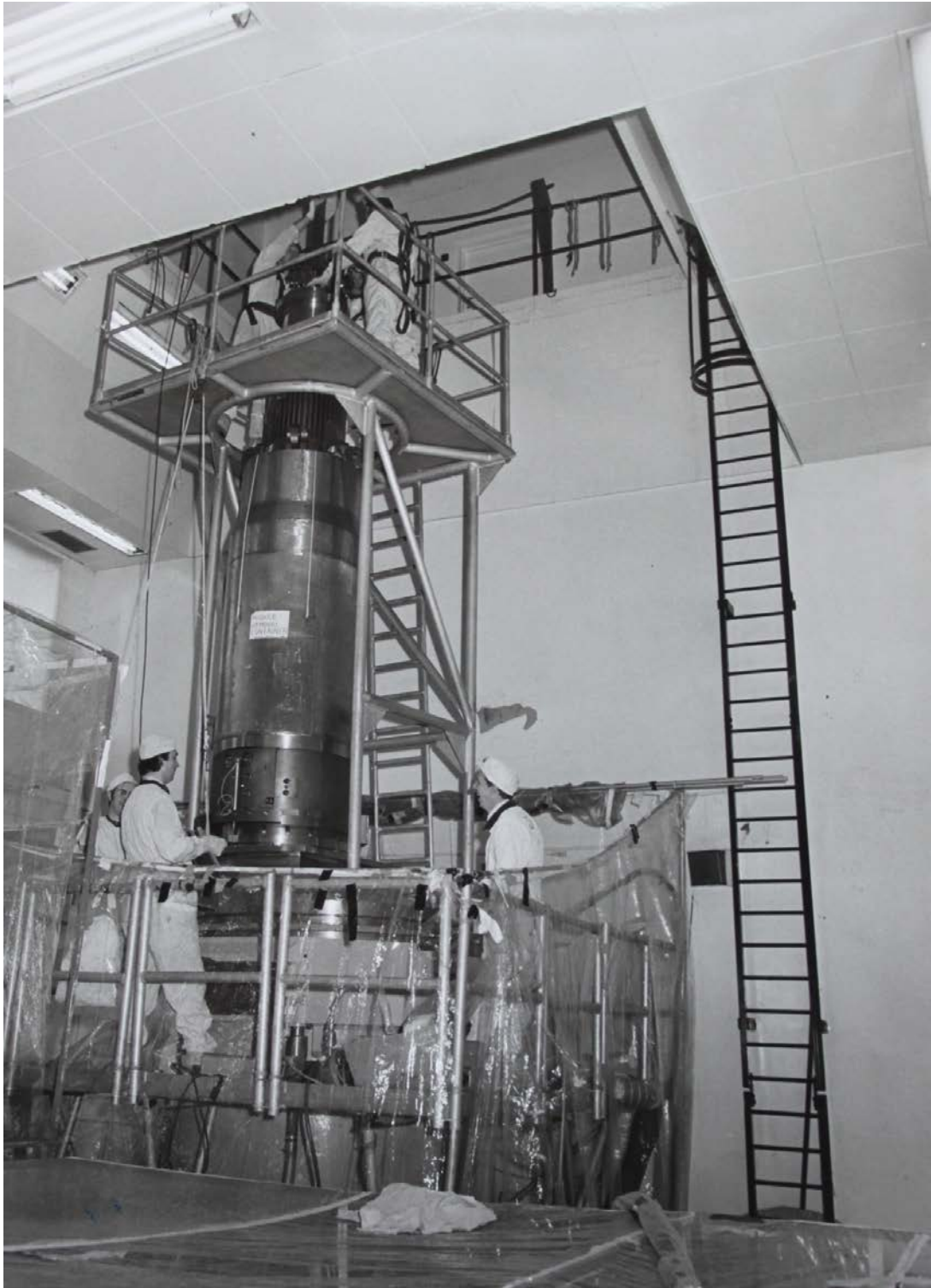
Figure 6.3: Workers in white overalls and cotton hats and gloves undertaking refuelling. The working conditions in this photograph are starkly different from all other images of work in the Dockyard. They are very clean and devoid of debris. Rather than dirty overalls, workers are all dressed in white. Source: RDL 2007.0008.22 PHA 11378 (black and white).
