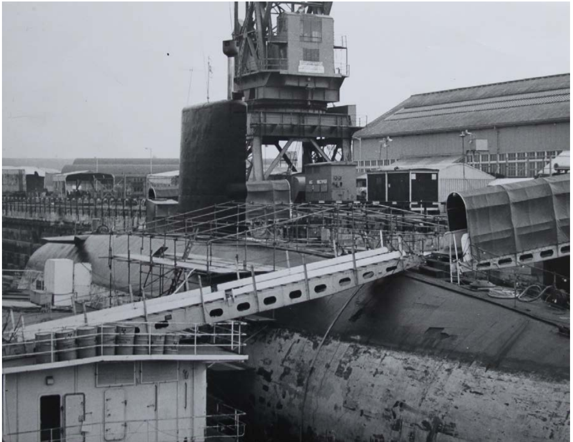
Figure 6.5: HMS Valiant in No 9 Dock 1 April 1968. Covered walkway to and from the submarine is visible on the right. Source: RDL 2007.0073.91 PHA 15347 (black and white).
