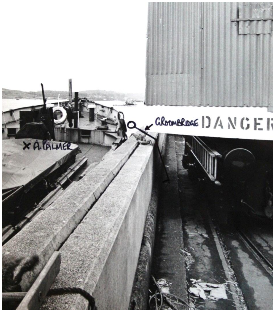
Figure 3.9: Injury to worker named Groombridge in 1973. The annotations to the photograph were added in pen, presumably by the person investigating the accident and suggest that Groombridge was injured by the crane and that A. Palmer was a witness. The angle of the crane housing suggests that it was turning (the crane travelled on rails, visible to the right of the photograph, but also rotated). Figure 3.5b shows the crane unloading bales from the barge, which may have been raw materials for rope making. Source: RDL Accident Photograph Collection (black and white).
