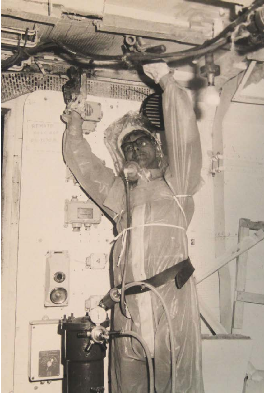
Figure 5.2 D Chandler, joiner, carrying out asbestos work using protective clothing and respirator. This photograph was printed in Periscope in August 1969 to publicise the protective measures that had recently been introduced. Compared to Harries' photographs, the work area in this image is remarkably clean. Source: RDL (black and white).
