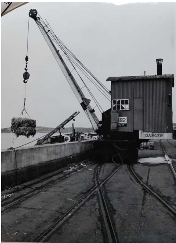
Figure 3.5a Travelling steam crane after the explosion of its vertical cross tube boiler on 4 July 1966. The corrugated iron that has been torn apart would have formed the cabin for the crane driver (see figure 3.5b below) and would also have housed the boiler. Source: RDL Accident Photograph Collection (black and white).
