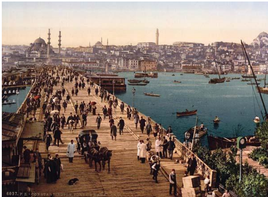
Fig. 16. Kara-Kevi Galata Bridge, Constantinople (1890-1900) Photograph, Private Collection
