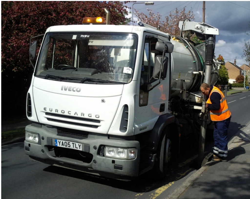
Figure 2.5 A gully pot being cleaned by an operative using the eductor truck.
