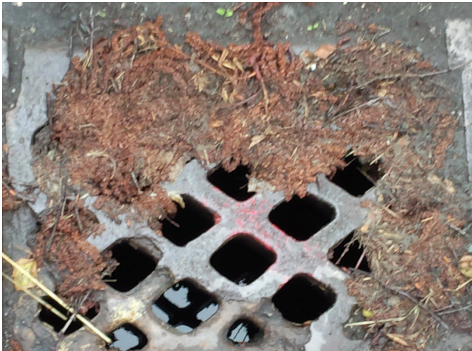
Figure 2.2 Detritus and leaf litter collecting on the diamond gully pot lid.
