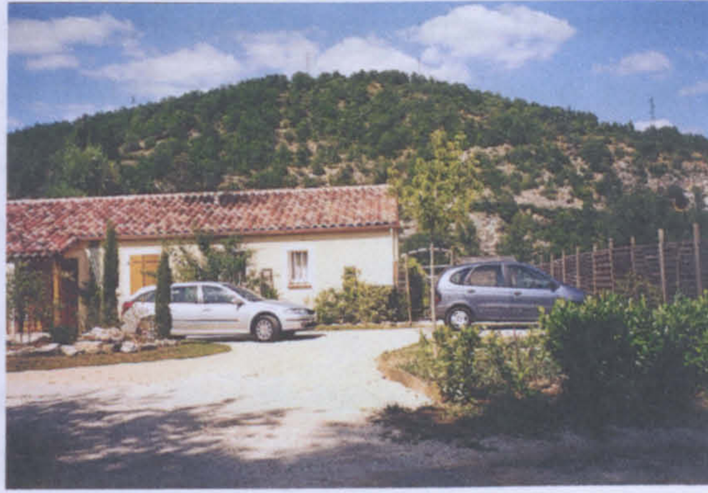
Figure 2.3: A newly built house
