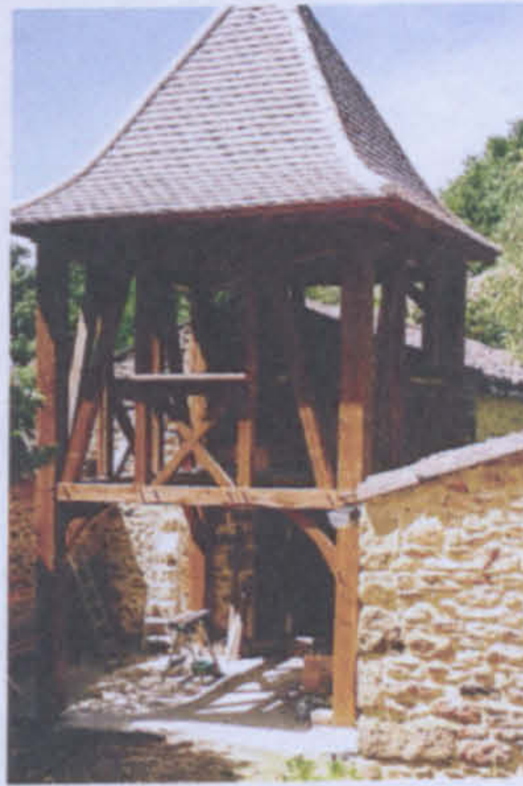
Figure 4.2: Daniel's Pigeonnier under construction
