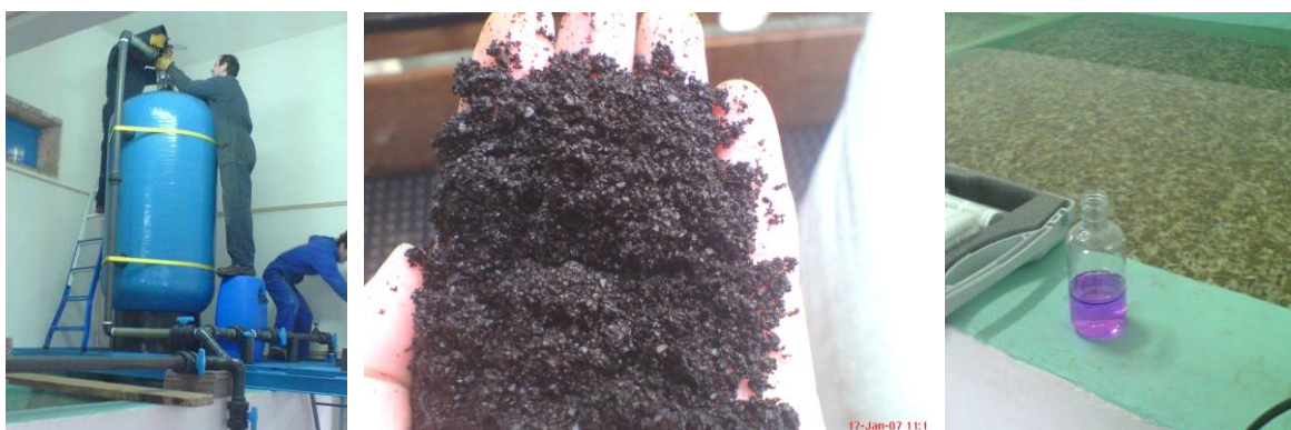
Figure 5. Installation of the reactive filter using iron oxide adsorbent medium.
