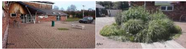
Figure 6.1: Before and after picture of the outlook of the frontage of the site featuring one of the raingardens.
