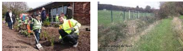
Figure 6.2: During the construction of the Swale and after.
