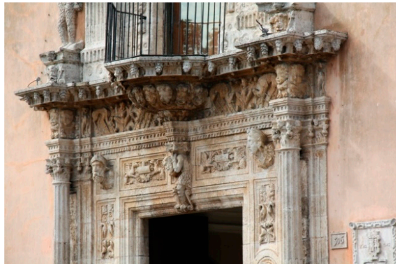
Figure 17. Detail, Lower Entablature and Dentil, Casa de Montejo. Photograph created by author.
