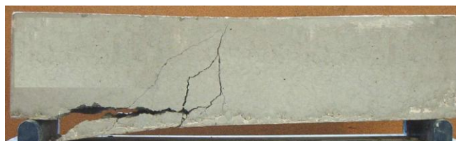
Figure 12: Delamination of the concrete cover.
