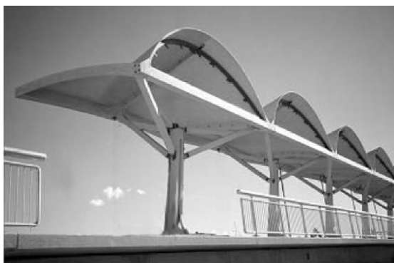
Figure 8. LRT Train Station, Shawnessy, Canada, 2003. Selfcompacting RPC. Shell thickness: 20 mm.
