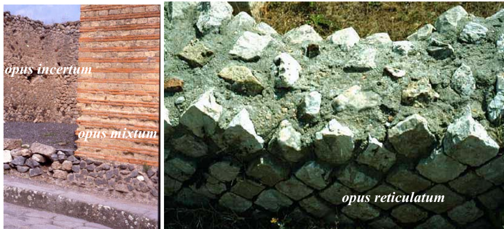
Figure 1. Roman concrete: opus incertum , opus mixtum and opus reticulatum .
