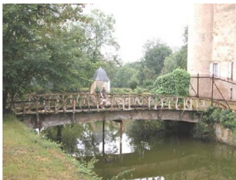
Figure 4. First reinforced concrete bridge, Monier, 1875.
