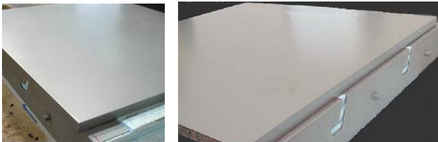
Figure 9: Application of the exterior aluminium finishing (left); retrofit module (right)
