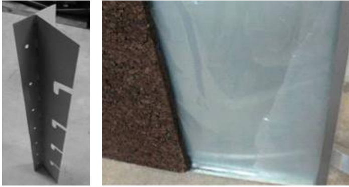
Figure 8: Support structure (left); smart vapour retardant and cork insulation application (right)
