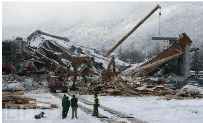
Figure 18. Bad Reichenhall ice-arena collapse
