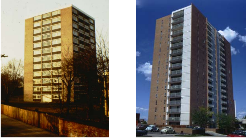
Figure 2 : Modern (unreinforced) masonry in high rise buildings, designed for compression and shear
