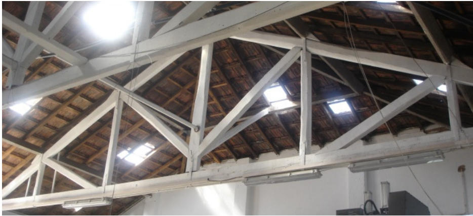
Figure 1 – Queen post truss analyzed
