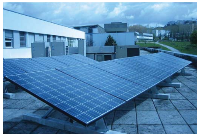
Fig. 8. Solar panel array installation
