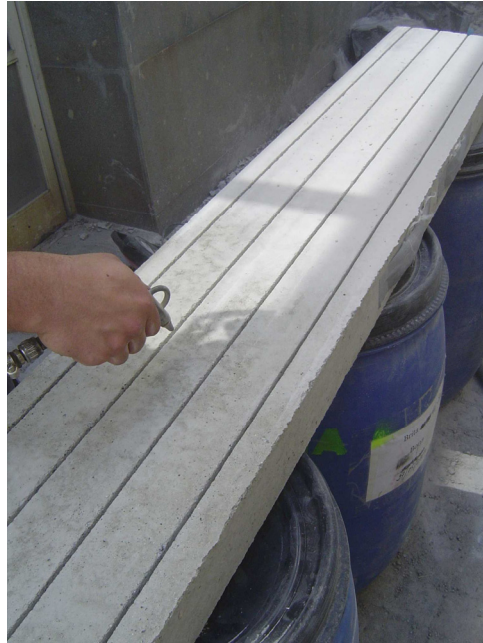
Figure 5.2 - Cleaning the slits using compressed air.
