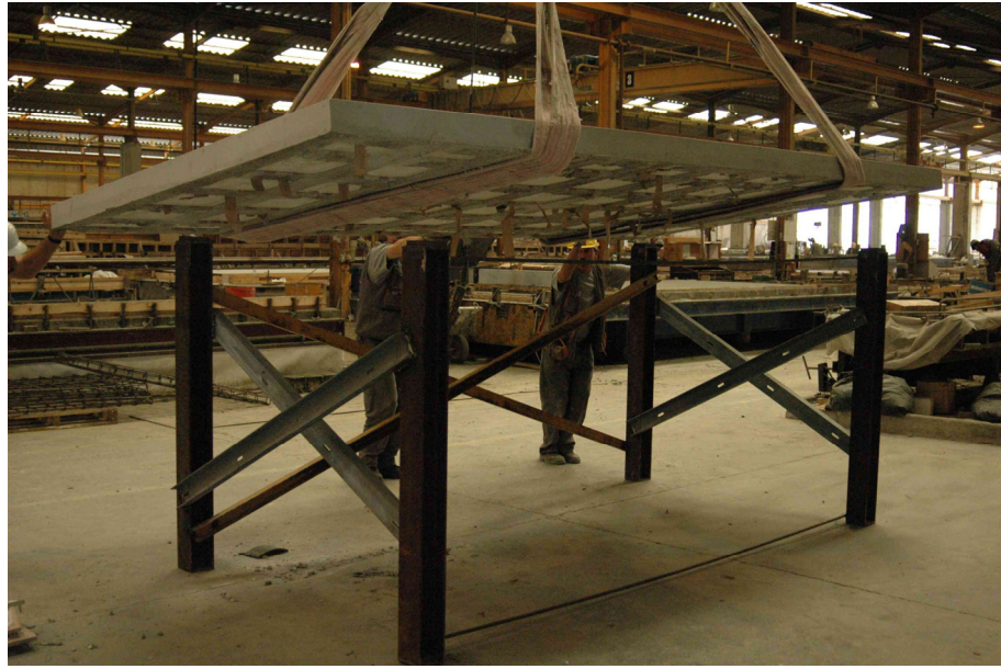
Figure 5.8: Placing the panel in the supports
