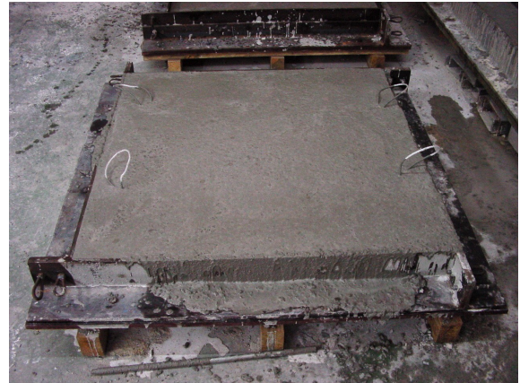
Figure 4.5: Panel after have been cast
