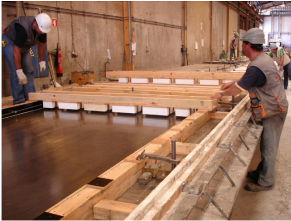
Figure 5.2: Placing the lightweight elements
