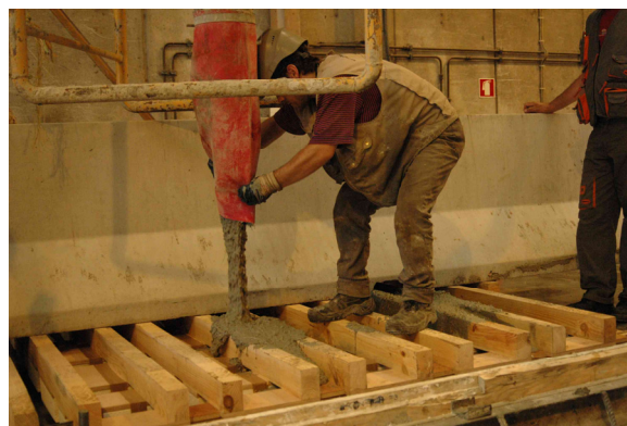
Figure 5.4: Casting the panel
