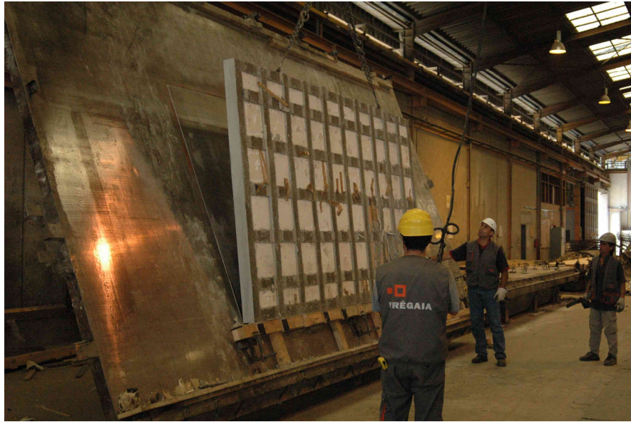
Figure 5.5: Demolding panel operations
