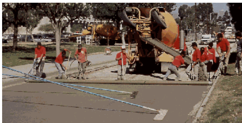
Figure 03 - Roller screed (revolving tube) for fixed-form paving on a street. [Photo: www.pavement.com ]
