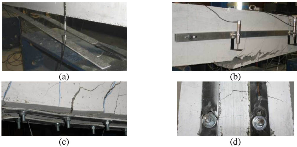
Fig. 4: Failure modes: (a) EBR beam; (b) NSM beam; (c) and (d) the MF-EBR beam.
