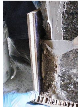
2. The damaged concrete cover was replaced by epoxy mortar
