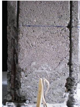
1. The too damaged concrete cover was removed
