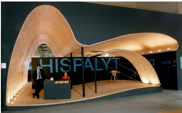
Figure. 2: View of the reinforced masonry shell system exposed in Spain
