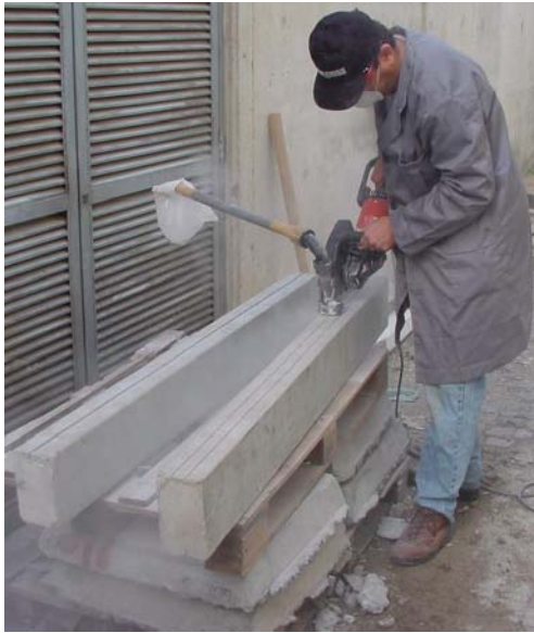
Figure 3. Sawing the slits.
