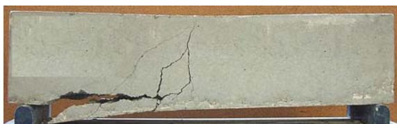
Fig. 17 Delamination of the concrete cover
