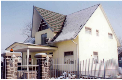
Figure 4.16. Bulzesc's family house
