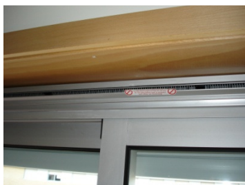
Figure 3.10. Ventilation grids on window frames.
