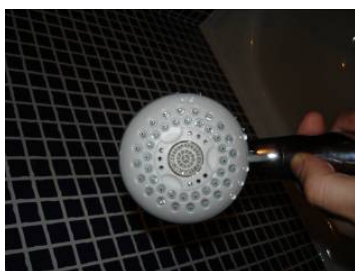
Figure 3.8. Low flow showers.
