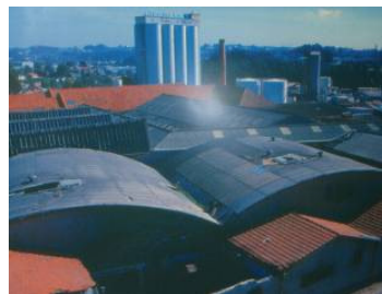
Figure 3.5. Aspect of the local before the intervention.
