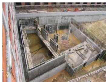
Figure 3.7. Rainwater tank (construction phase).
