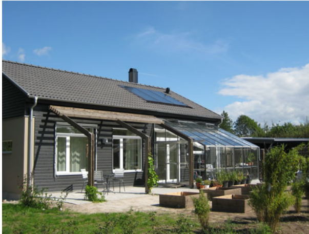
Figure 3.19. External view of the of the Villa Trift single family house (case study).
