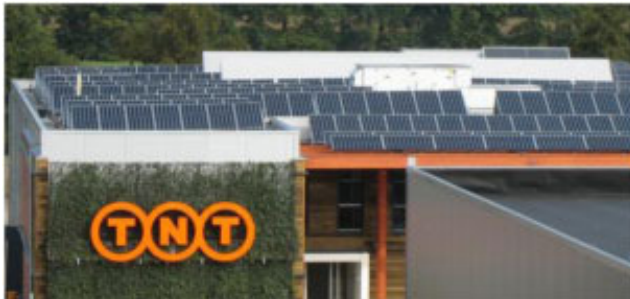
Figure 3.25. The electricity is generated by 300 PV panels on the roof
