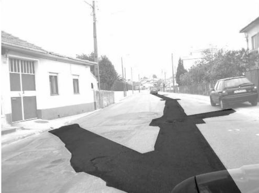
Infrastructure does not contribute to the improvement of spatial quality
