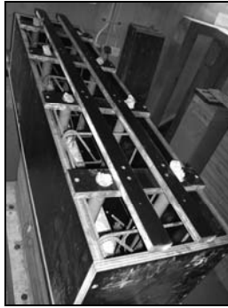
Figure 4.11 – Construction of the reinforced concrete top beam.
