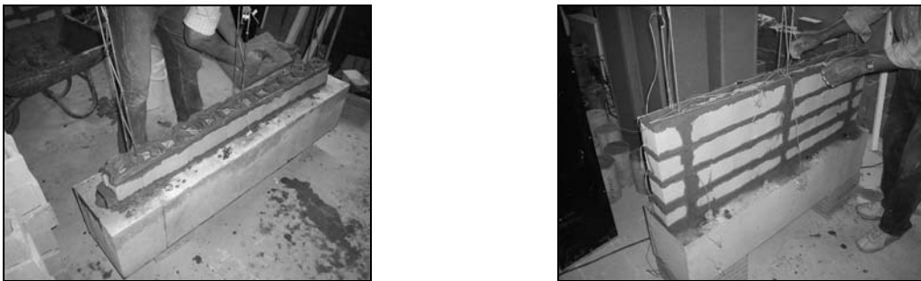
Figure 4.9 – Construction of the walls.
