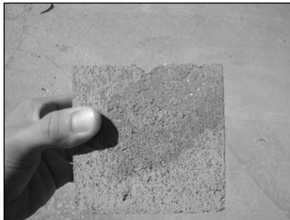
Figure 3.4 – Damages in half blocks of 2C-units.
