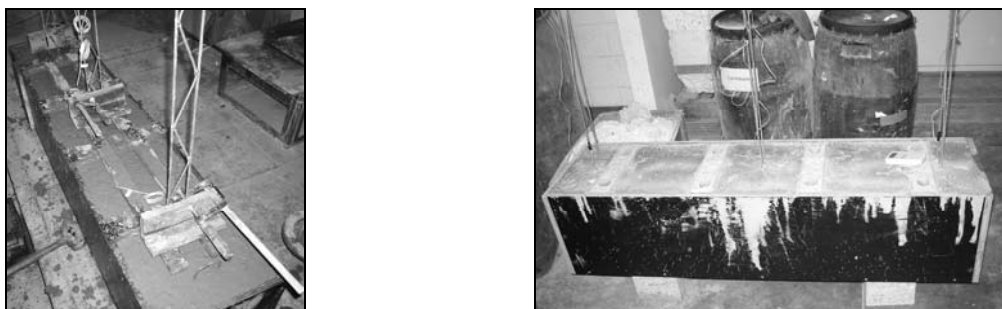
Figure 4.8 – Construction of the bottom reinforced concrete beam.
