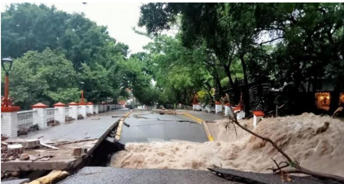
**IMAGEN 5.0 Derrumbe puente vehicular**
