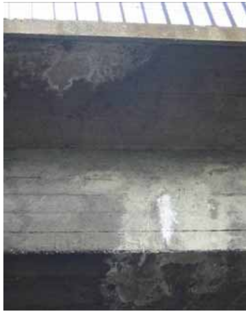
Fig. 5-6 Example of leaching effects – lime bloom (photographed by Author)
