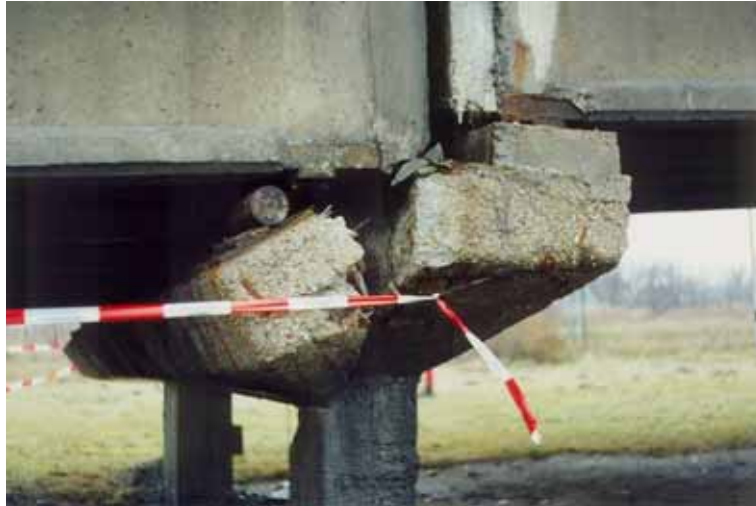
Fig. 5-14 Example of effects of overloading (photograph courtesy of Kazimierz Bieniek, WUT)
