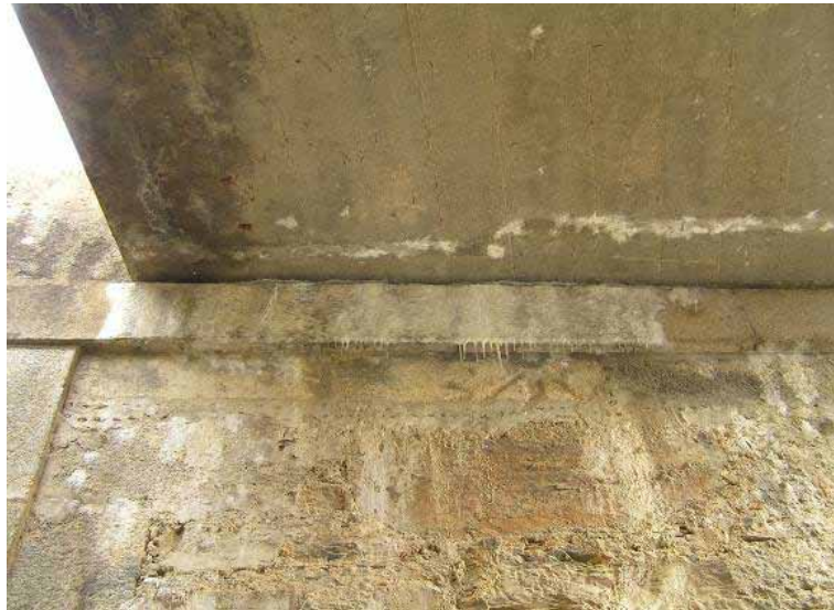
Fig. 3-2 Example of contamination of concrete (photographed by the Author)
