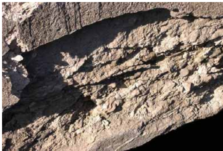
Fig. 5-12 Example of the result of freeze-thaw action (photograph courtesy of prof. Jan Bień, WUT)
