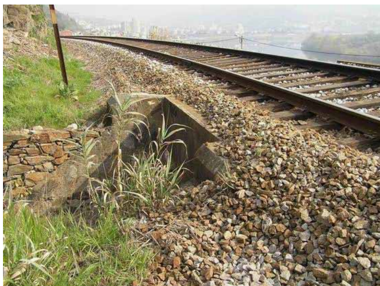
Fig. 2-15 Example of railway track with ballast (photographed by the Author)
