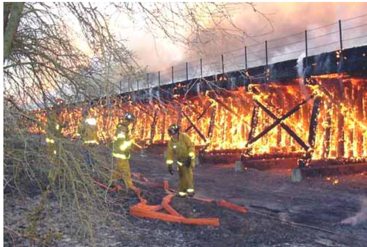
Fig. 5-11 Example of influence of high temperature mechanisms (fire of the Sacramento Bridge USA) – picture downloaded from http://www.uprr.com/newsinfo/2007/sacramento_bridge.shtml
