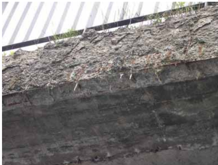
Fig. 5-18 Effects of weathering (photograph courtesy of prof. Jan Bień, WUT)
