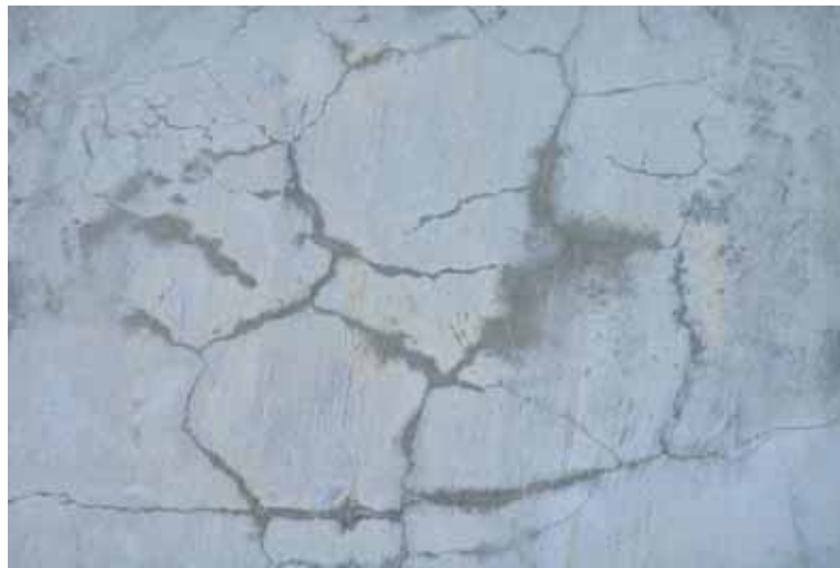
Fig. 5-2 Effects of alkali-aggregate reaction (photographed by Author)
