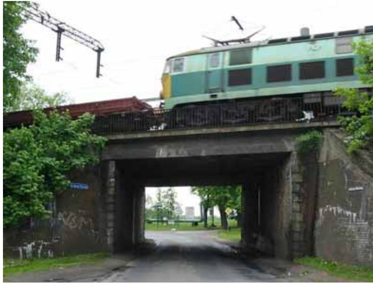
Fig. 2-12 Example of slab span with rectangular cross section (photographed by the Author)
