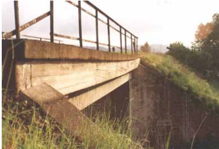
Fig. 5-8 Example of effect of creep (photograph courtesy of Zygmunt Kubiak, PKP)
