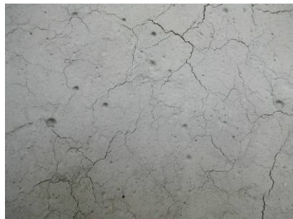
Fig. 5 – Concrete surface appearance at the beginning of the cooling process
